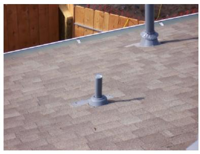
7. There was a neoprene seal that was improperly positioned over the utility room. This seal will hold water and leak in the future.
