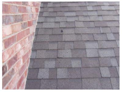
9. Nail holes existed in the roof over the north side of the garage, which will leak. These shingles should be replaced.
