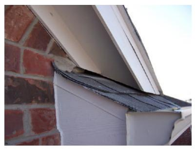
1. There was no head flashing at the eyebrow section of roof at the front gables, including at the front of the garage. Additionally there were large gaps in the cornice work, which can allow animals access to the building.
