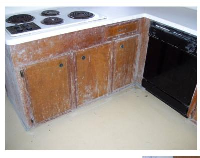
19. Mildew could be observed on many of the finished surfaces at the interior of the building, indicating a higher than normal humidity at the interior of the building.
