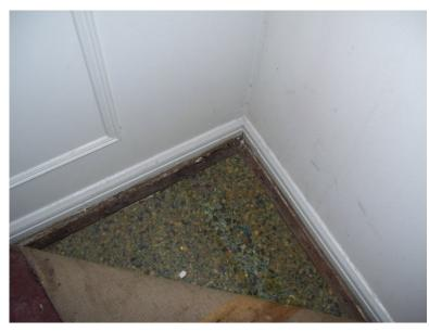
15. Evidence of water entry, past or current, was observed at several locations, including at the north side of the living room, as indicated by stains in the tack strip and carpeting along the north wall; at the dining room, as indicated by stains in the tack strip along the north wall; and at the north bedroom at the northwest corner of the room, as indicated by stains in the tack strip.
