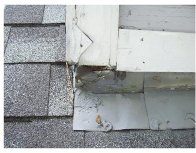
3. The flashing installation at the front dormer was improper where the top edge of the head flashing was visible. This will allow water to bypass the flashing at this location and run into the structure of the building.
