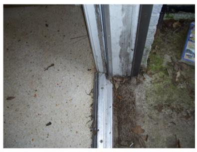
21. The threshold at the entry porch appeared to be at or above the floor height at the entry foyer. This may allow water blowing onto the front porch to run in around the entry door threshold and may be difficult to repair due to its configuration.
