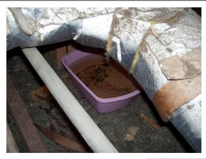
1. Catch basins were noted in the attic at possible points of roof leakage. The catch basins may or may not be necessary at the current time. They may have been necessary before repairs were made.
