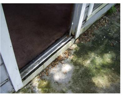
6. Vulnerability to termite infestation was observed where siding was in contact with a concrete surface that is not monolithic with the foundation. Subterranean termites can enter the structure below or through the siding without being observed.
