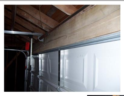
16. Panels at the overhead garage door were bent or damaged at some locations, which may require replacement of sections of the door in order to improve its appearance to a normal condition.
