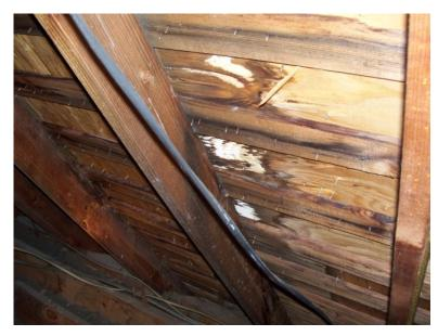
4. The roof decking was deteriorated below the southwest corner of the upstairs dormer adjacent to the center bedroom. There is evidence that the flashings at this location may not be well fitted and may be the cause for evidences of water penetration at this location. A catch basin full of water located below this area indicates that leaks through the roof may be active in some areas.
