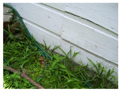
18. Siding along the west side of the garage did not appear to lap the edge of the foundation. This creates a potential for water running down the siding to run onto the foundation and into the garage if not corrected.
