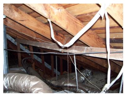
7. Vertical bracing normally used to support the mid span of the roof rafters did not exist where the warm air furnace had been installed.
