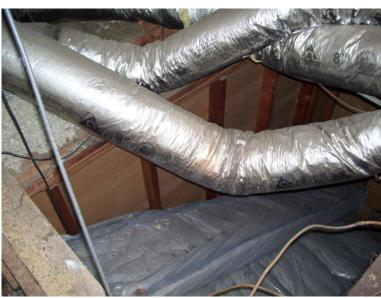
12. The attic insulation was observed to be missing or out of place at the den, at the vertical walls at the south attic and at the attic over the stairs, which can result in loss of energy.
