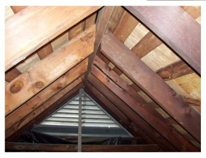
9. The ridge beams were not wide enough to support the entire width of the miter cut on the end of the roof rafters. Even though this is a common observation, the greatest strength requires that the ridge beam be wide enough to uniformly distribute the roof load across all the width of the rafter miter cuts.
