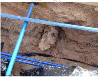
9. A tree root had not been sufficient cut off at the south grade beam allowing it to extend into the grade beam reducing its effective width. The root should be cut at the face of the beam.
