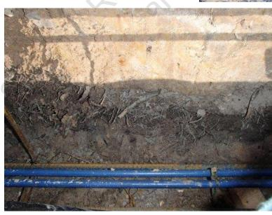
12. There was a layer of organic material observed between the virgin soil at the site and the fill soil which appears to be the original forest floor. The observed debris included braches and leaves. This material should have been removed before placement of the fill because it may result in differential movement of the building's foundation in the future.
