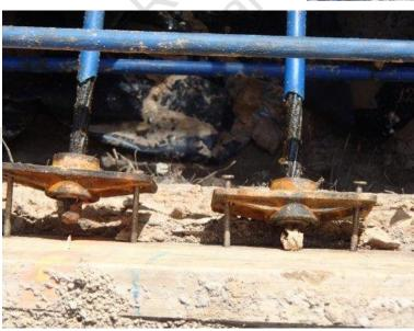
3. The fixed ends of the reinforcing tendons were in contact with the forms. The cables should be installed hung against forming nails to ensure a minimum of 3/4 inches between the ends of the tendons and the surface of the finished concrete. Failure to properly install the cable ends can result in corrosion failure of the anchor point, leaving a portion of the foundation without sufficient reinforcement.
