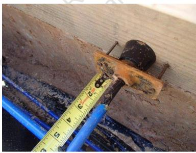
6. The protective sheathing had been excessively cut away from the tendons at the anchors to allow installation of the cables through the anchor points, leaving a portion of the tendons exposed. No more than one inch of the cable should be left exposed. The sheathing should be repaired to prevent bonding between the concrete and cable as the concrete cures, which can prevent proper tensioning of the cables.
