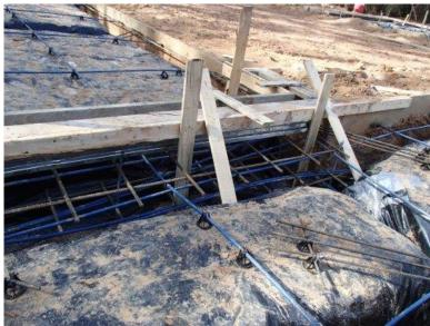
10. The installation of the metal keyway detail at the narrow section of foundation between the house and the south garage was incomplete and should be completed in accordance with the specification detail. It appears this may require resetting of the steel pin bars.
