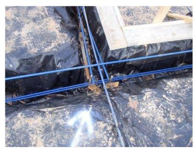
13. The dead ends of tendons terminating inside the forms were set too high and should terminate in accordance with the plans which appears to specify the at the interior of the beams.
