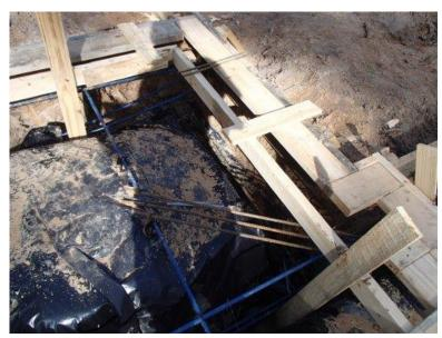
16. Reinforcing steel was missing in the forms at some locations where it was specified at the beams, including at the north side of the building. The steel should be placed in accordance with the plans.
