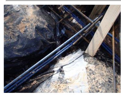
4. Plumbing lines occupied the bottom of grade beam trenches and affecting the proper placement of the reinforcing cables. This may affect the performance of the cables and their ability to provide sufficient reinforcing to the beams.
