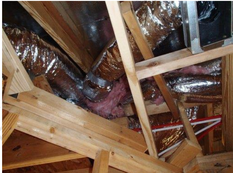
24. The liquid line connection at the evaporator coil was left open and facing upward. This creates a greater potential for contamination to enter the liquid line and could cause damage to the thermal expansion device inside the coil.
