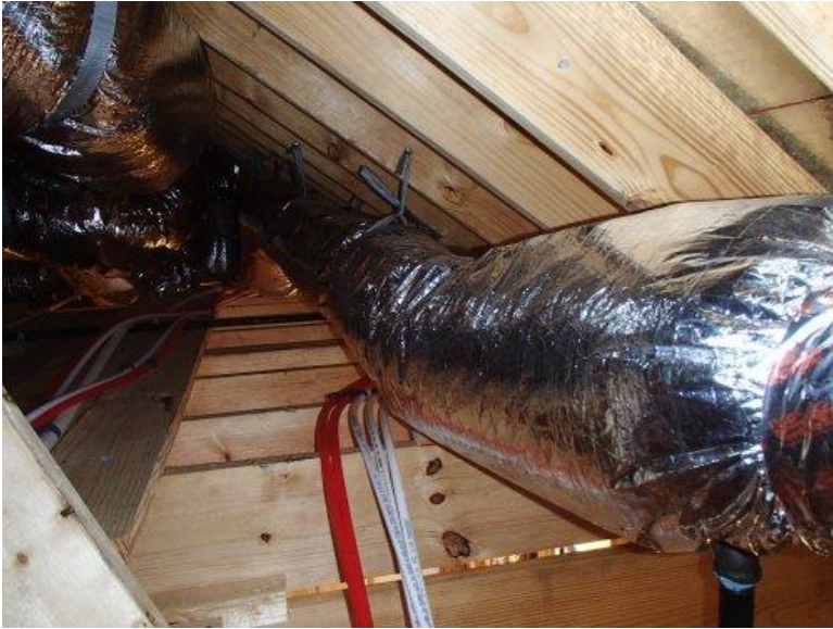
23. Ductwork was compressed together in the attic space over the master bedroom and master bathroom. Compressed ductwork has a greater potential to sweat and reduces energy efficiency.
