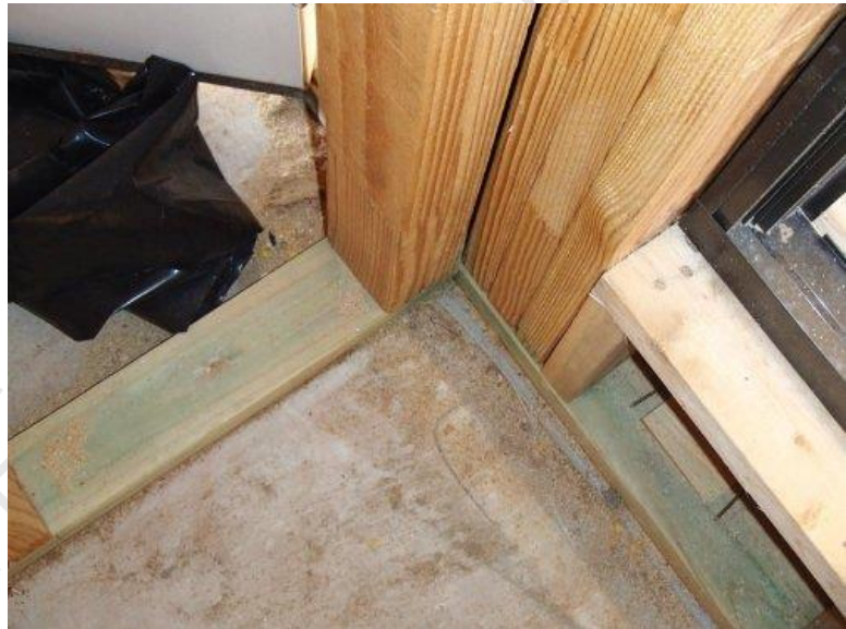
30. It was indicated that the curb along the north end of the living room balcony was to be removed, requiring modification of the balcony dry pan.
