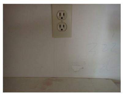
13. Evidence of water entry, past or current, was observed at the quarters' microwave oven cabinetry, as indicated by water streaks below the outlet; at the quarters' living room, as indicated by stained carpeting; at the enclosed porch glass walls and south partition wall addition; at the west wall of the living room at the fireplace, as indicated by a seam bulge; at the fireplace firebox, as indicated by mineral {...full text in report}
