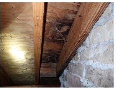
3. You should make further inquiry as to the status of the following observed evidences of roof leaks, current or previous: decking stains at the hall bathroom; seam bulges in the living room; sheetrock patches in the master bathroom closet; rotted decking at the fireplace in the attic; and stained fascia at the east side of the northeast bedroom as viewed from the attic. You are cautioned that other {...full text in report}
