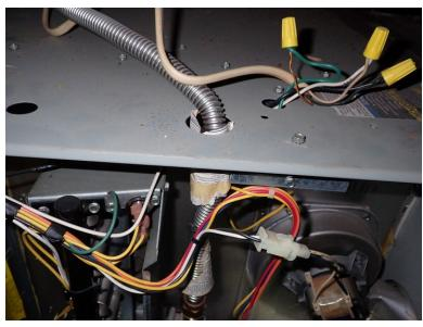
21. Flexible gas coupling was routed into the north zone furnace case. Most codes do not allow flexible coupling to extend inside the case as it is a fire hazard. The gas control valve should be hardpiped to the outside of the case, where flexible coupling should then be attached.
