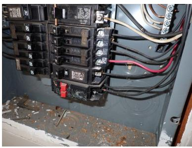
9. Two breakers were observed that appeared to serve a single conductor in the garage sub panel box, indicating that conductors may exist that are wired as a 240-volt circuit without appropriate ganging of the breakers serving the conductor to ensure that both legs of the circuit trip. This is sometimes performed to serve kitchen appliances which can share a common neutral power to a{...full text in report}
