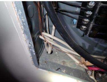
6. Wires had been run through openings in the study closet panel box that did not have strain relief and did not fill the openings to prevent a fire starting at the panel box from spreading to the structure.
