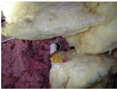
15. It was observed that the south zone air conditioner primary condensate drained into a dedicated trap. Careful observation of this dedicated trap is recommended to ensure that it does not dry out in the wintertime when the air conditioner is not used and allow sewer gases to be drawn back into the conditioned air stream. Further, algae may form in the drain trap, causing the drain to overflow. {...full text in report}
