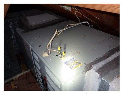
1. Electrical wire splices that were not in junction boxes were observed in the following locations: at the attic, at the north air handling unit, and at the attic over the dinette.
