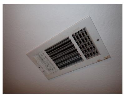
13. Mildew could be observed at diffuser outlets in the rooms, including at the quarters' bedroom and at the quarters' kitchen. This can indicate sweating of the diffuser grille due to air infiltration at the register box and, in some cases, may indicate a negative pressure created by poor balancing or a lack of adequate ventilation air. This should be investigated by an HVAC contractor.
