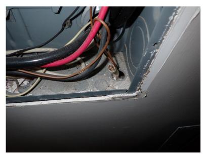
4. Wires in the study closet breaker box were observed to be improperly terminated.
