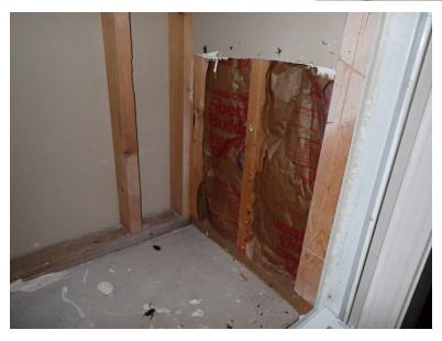
12. Batt fiberglass insulation could be observed in the north zone air conditioning return chase. This is considered unacceptable since this could result in insulation contaminating the air stream, allowing it to be distributed in the zone through the registers. The inside of the chase should be covered with drywall wall coverings or the insulation should be removed.
