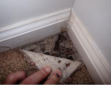
3. High moisture readings and evidences of deterioration in the finishes could be observed at the base of the wall at the master bathroom closet adjacent to the shower. The source for moisture causing high moisture readings and deterioration was not determined. Further inquiry of the owner to provide history of repairs at the shower is recommended. Investigation may require removal of wall coverings {...full text in report}
