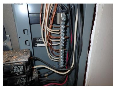
8. Wires had been run through openings in the garage sub panel box that did not have strain relief and did not fill the openings to prevent a fire starting at the panel box from spreading to the structure.
