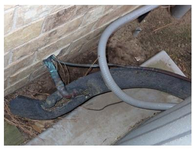
9. Some foam insulation was torn off the refrigerant return line near the north zone condensing unit. Some energy will be lost as a result of the missing insulation. In newer construction, a protective covering is required on the insulation.
