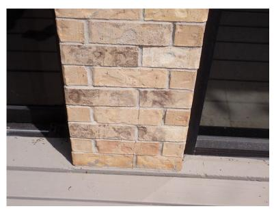
10. Cracks could be observed in the brick veneer at the base of the columns at the back porch. The configuration of the cracking observed may indicate woodframed structure inside the columns that was in contact with the masonry and has become wet, causing it to expand and split the brick veneer. Further investigation is recommended and would require removal of brick veneer for inspection as water{...full text in report}
