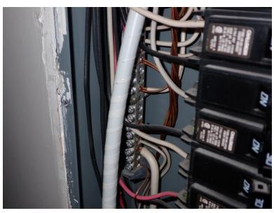
3. Neutral buss connections were made with more than one wire attached at each set screw at the study closet panel box. Normally, only one wire (circuit) is connected to each buss terminal opening. In some cases, this can require expansion of the buss.
