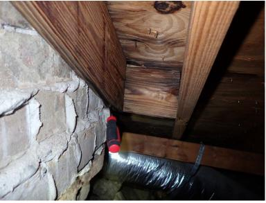
12. Trusses had been constructed to support the midspan of the roof over the area of the garage nailed to the sides of the ceiling joists. Site-built trusses often do not perform as well as engineered trusses, and some of the connections were starting to separate, although the roof structure appeared to be performing satisfactorily. The trusses should be monitored and reinforced if the connections further {...full text in report}
