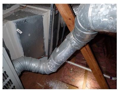
22. The north zone vent flue pipe appeared to be pieced together from segments with poorly made joints and evidence of leaks in at least one joint. This should be investigated by an air conditioning contractor who can repair or replace the flue as necessary.
