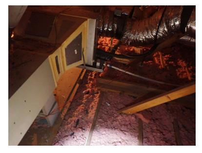
18. There was no service decking provided to service the south zone evaporator coil, which creates a hazard.
