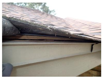
6. The roof deck did not extend to the fascia boards along the lower edge of the roof, leaving a gap. The drip edge flashings were installed resting on the fascia boards rather than properly extending up the deck of the roof as required by current construction code. This allows the drip edge to lay horizontally, which could allow water running off the edge of the roof to be directed into the eaves and may be related to evidences{...full
