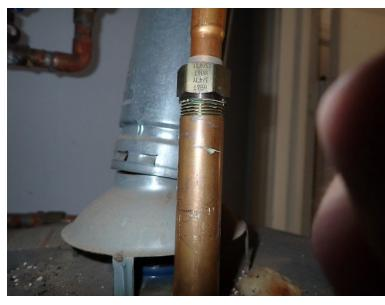
6. The hot gas vent pipe was not properly connected to the garage water heater draft diverter. Combustion products may be emptied into the building.
