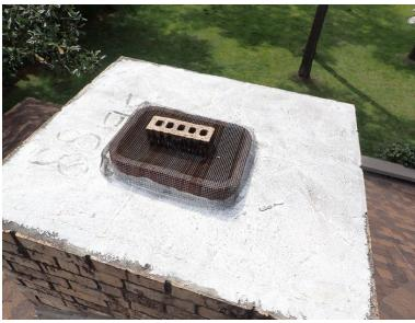
9. Sealant had been applied at the cap at the fireplace flue chase where it had developed cracks. There were evidences of water penetration at the interior of the building, indicating past water penetration through the cap. The sealant may be a temporary repair, and this should be investigated by a chimney sweep.
